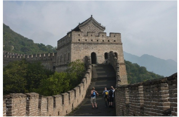
the Wall of China
